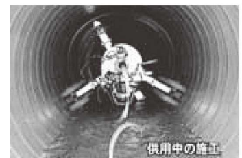
[管路施設長寿命・耐震化]
